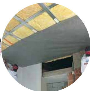
4. Namestimo parne ovire ( s_d \approx 2 \text{ m} ) ali parne zapore ( s_d \geq 100 \text{ m} )
